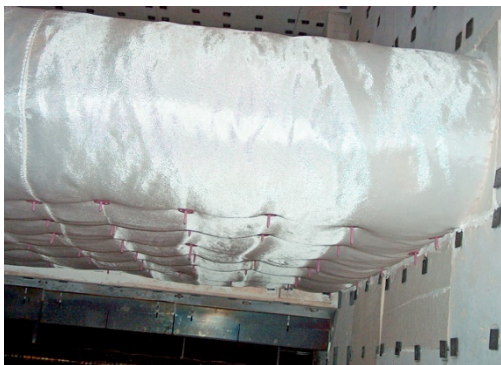
Typical design Refrex® Expanchor® Lining system:
